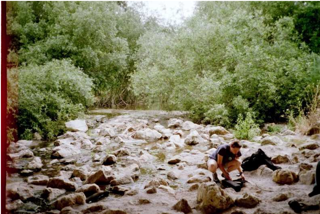
Figure 3. At Atascadero at Patterson Avenue (AT2) a concrete and rock apron leading under the bridge acts as a weir and forms a long, narrow impoundment which can be seen in the middle of the photo. In summer, water trickles from the pond over the rock apron. At around 11 AM on August 2005 (the photo was taken in June) dissolved oxygen in the ponded water had a concentration of 4.6 mg/L; ten feet downstream the concentration had increased to 9.1 mg/L.
